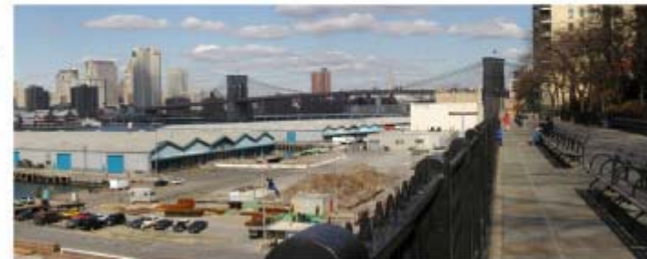
Esplanade over Highway
